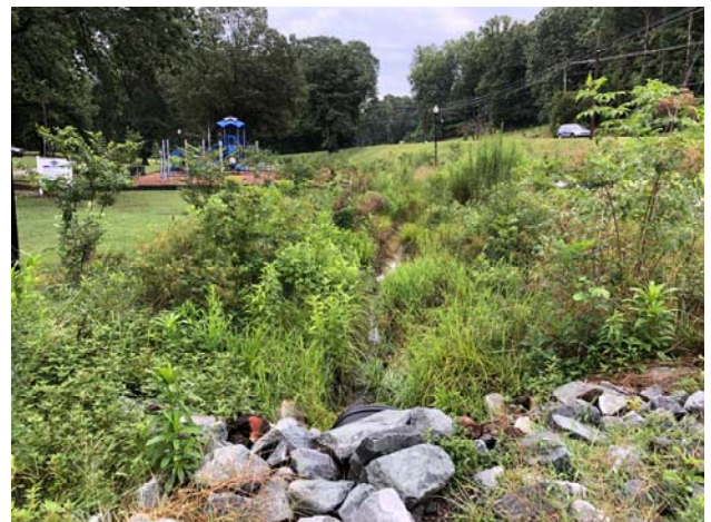
Green lush after water control structures with erosion halted.
