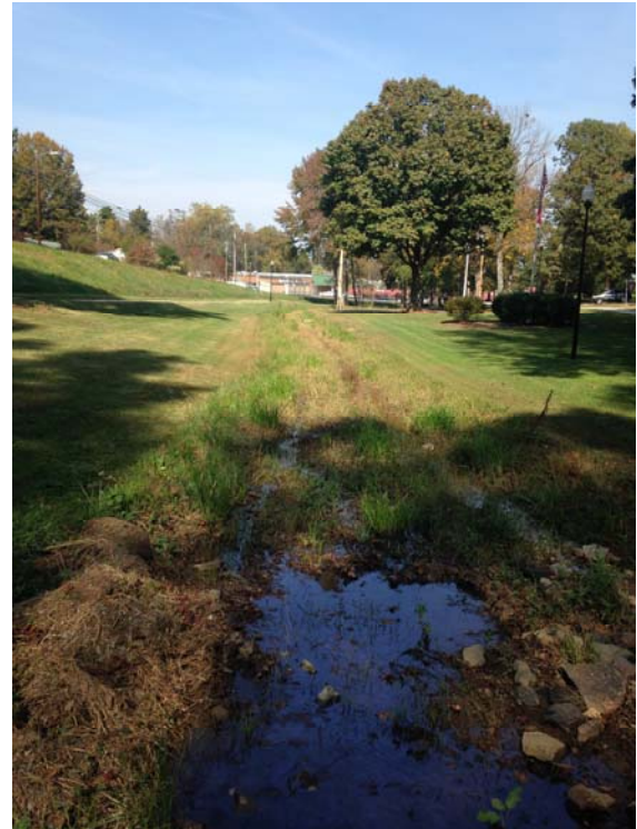
Park before, erosion with each rain..
