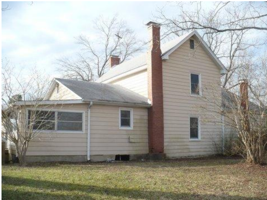
East side of building
