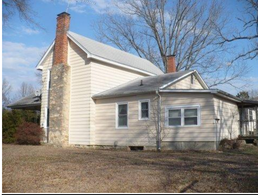
West side of building
